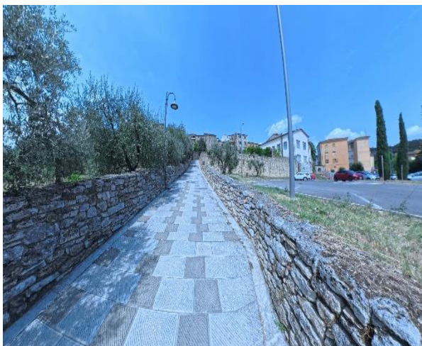
19 First section of the path
